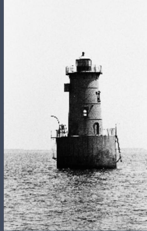
*Sharp's Island lighthouse, slightly tilted in de Gast's photo, took a much more noticeable, fifteen-degree list when ice and tides canted it in the winter of 1977. Despite its precarious angle, it remains an active aid to navigation.*
